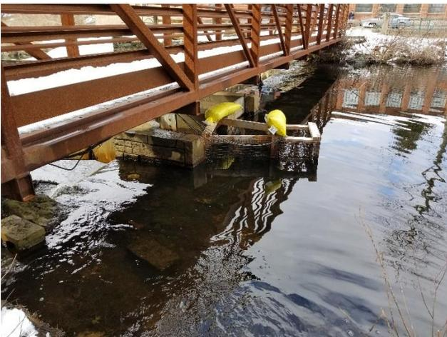
The fish counting weir at the exit of the Jordan Brook Fishway in Waterford. The fishway, located at a Town Park, has a new signboard this year, worth checking out.
