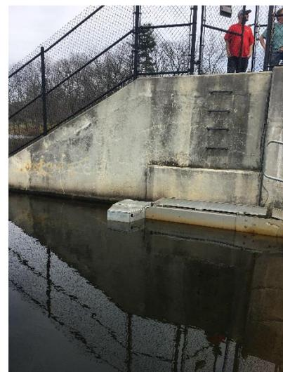
*The exit of the Bunnells Pond Fishway on the Pequonnock River in Bridgeport. This is the top end of what may be the tallest steepass fishway in the region. The spillway is to the right. The lighter silver box at the end of the fishway is the housing for our video camera. Images are analyzed by our partners at the Beardsley Zoo and streamed on-line. We'll share that link with you in a future report.*
