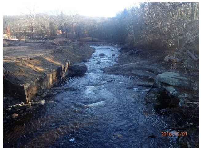
Norton Mill Dam after removal and some fall rains. The mill building has been razed. Note same rock outcrop to the right. The liberated stream channel is once again a bedrock rapids with very little soft sediment.
