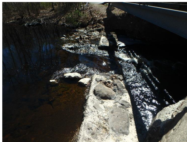
The dam as it looks this spring. A nice smooth tongue of water flows through the notch allowing fish from Hallville Pond to swim up through the notch and into Straight Pond and beyond.
