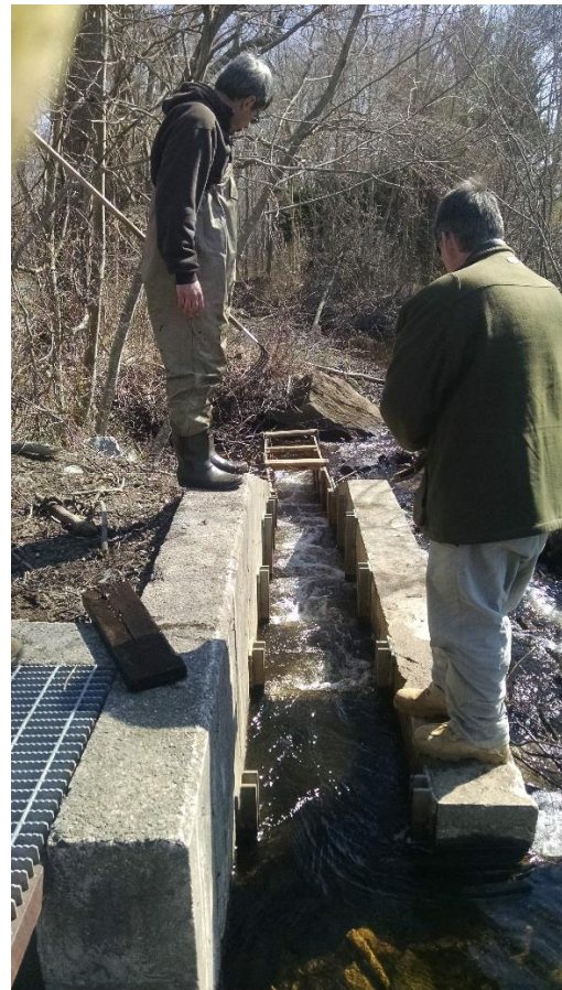
Chalker Millpond Fishway in Old Saybrook didn't operate much last year due to beaver dam problems. The beavers are now gone and we opened the fishway yesterday. Bruce Williams and Tim Wildman look on.
