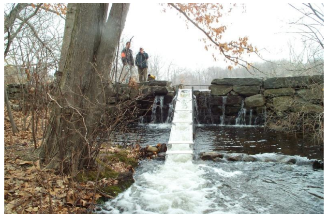
Perhaps the smallest fishway in CT: The Hummers Pond Fishway on Fence Creek in Madison started life as one of our earliest ones made out of wood but replaced with aluminum. It gets a call out this week because it appears that a wave of alewives have gone up it this past week!
