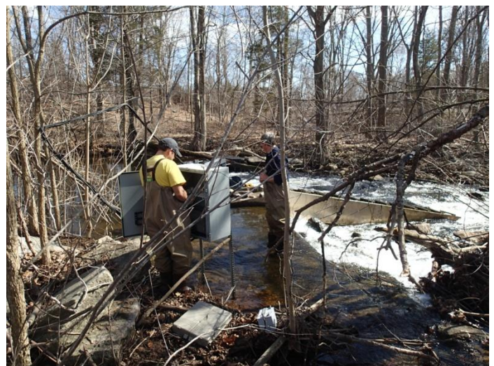
Fish Counter at Landon Dam: Dave Ellis and Bruce Williams (partially obscured by branches) install a fish counter at the Landon Dam fishway.
