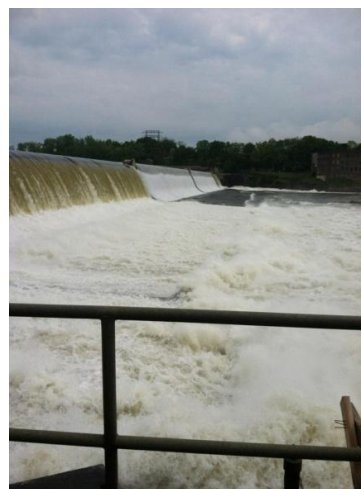
When there is a lot of water pouring over the Holyoke Dam, they cannot operate the fishlift. That is currently the situation. Once the flows drop down to below 40,000 cfs, lifting will begin. Once fish start passing Holyoke, upstream fishways will begin to be opened.
